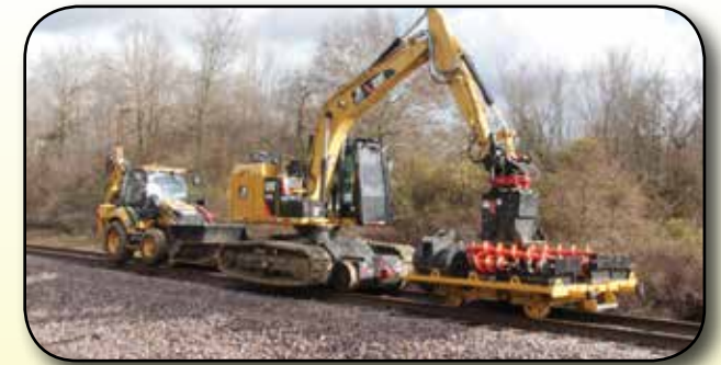
Hi-Rail to culvert area
