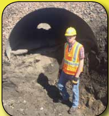
Large culvert with packed in mud and debris
