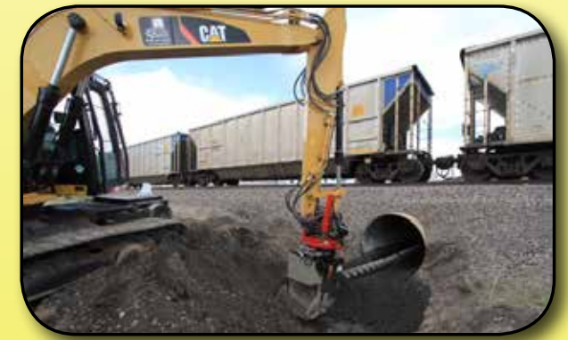
Work is done off-track
